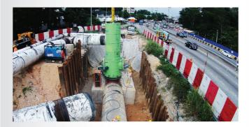
Under-Pressure Technology Line-Stopping are means of temporary isolation on the pipeline. This has proved effective in areas where valves are unavailable for maintenance, relocation of pipelines and emergency situations. With the proper solution and bypass, work can be carried out in the pipeline without the interruption of water supply.
