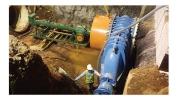
Under-Pressure Technology Hot-Tapping is carried out to core a hole in the existing pipeline without shutting it down. The tapping can be used as a branch off for a new pipeline or for line stopping purposes.
